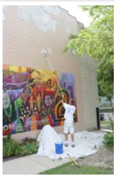
▲ House of Peace site: The painter covers spots in preparation for another coat.
